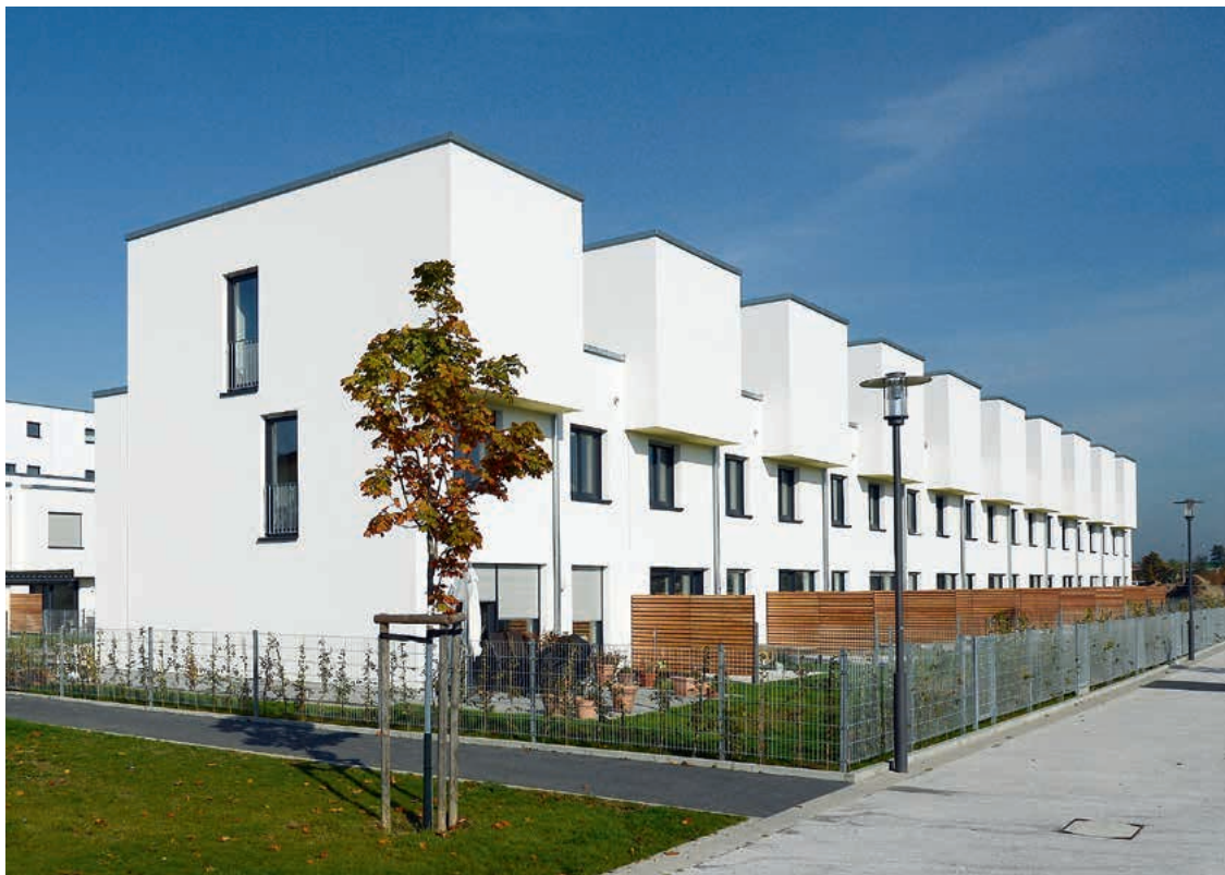
Neubau Centro Verde (Neckarstadt-Ost)
